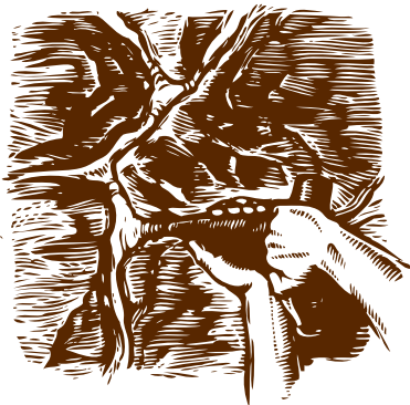
FIG. 7 Grout Joints
